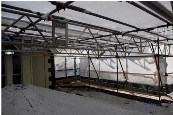
Figure 1 Scaffolding and temporary roof installed – 29.05.2015 (JGA)
